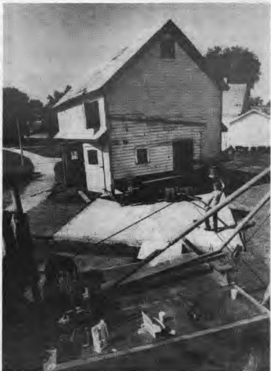
Workers place the 96-year-old building on its new foundation.
