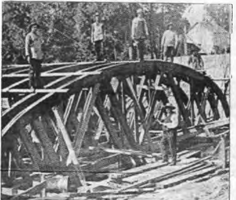
A concrete bridge over the Des Plaines River at Dundee Road under construction in about 1920. It is still used today.
