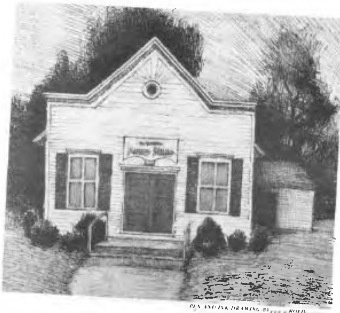
Original Village Hall
